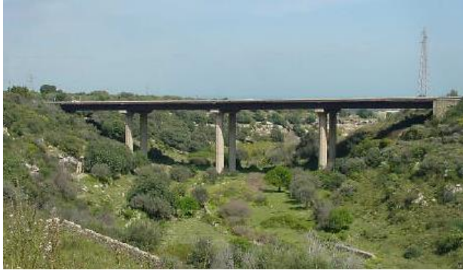
Figure 2 West side elevation of the bridge (Protezione Civile, 2019)
