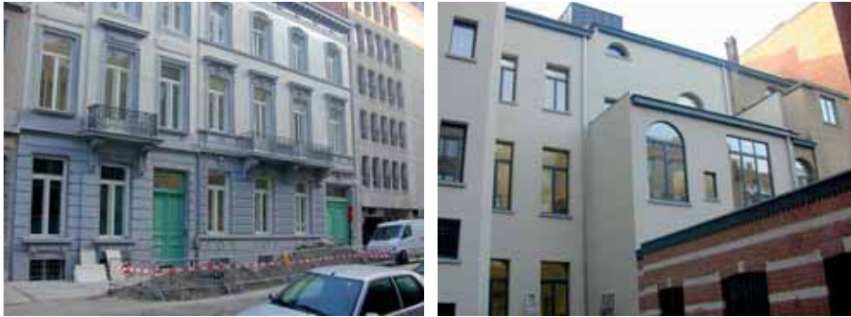
Figure 4: Front and back façade of the renewable energy house, Brussels, after refurbishment. Source: Adapted from New4Old [27].
